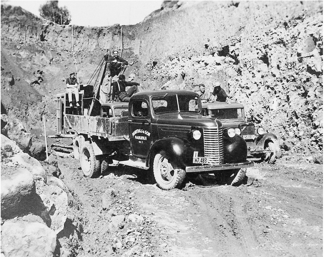
Thirteen thousand cubic yards of spoil was taken out of this huge cutting known as the "False Top" situated just below the Waituhi Saddle. Beautrais & Son used a 10RB excavator (rear) and International trucks to remove the spoil. The huge boulders at left were rolled over the bank.
