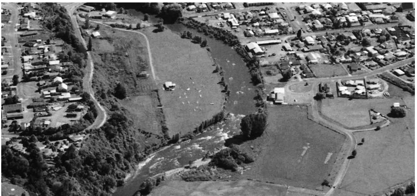
According to stories passed down to local identity Mere Bell by her grandmother, Okeroa Te Turi (wife of Te Huia Pikikotuku), the area originally known as Taumarunui was the flat area below Te Peka (shown above) which stretched downstream from the present road bridge to the point opposite Cherry Grove and before the Ongarue River junction. Mrs Bell was also told that the Maori chief, Maru the Great, was killed in battle on the big rock that used to sit in the last long rapid in the Ongarue River about 100 yards above the junction (centre foreground). This is basically the reason why the river flat above this rapid was known to the Maori as “Taumarunui”.
