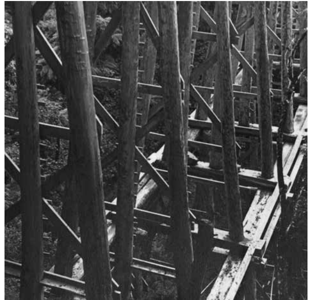
ABOVE: Parts of the top layer of the “double-decker” can be identified. The three uprights are called “legs” and the top cross member is the cap and the three together (with the cap) is called a set. That upon which they rest is the sill with the braces being the X.
