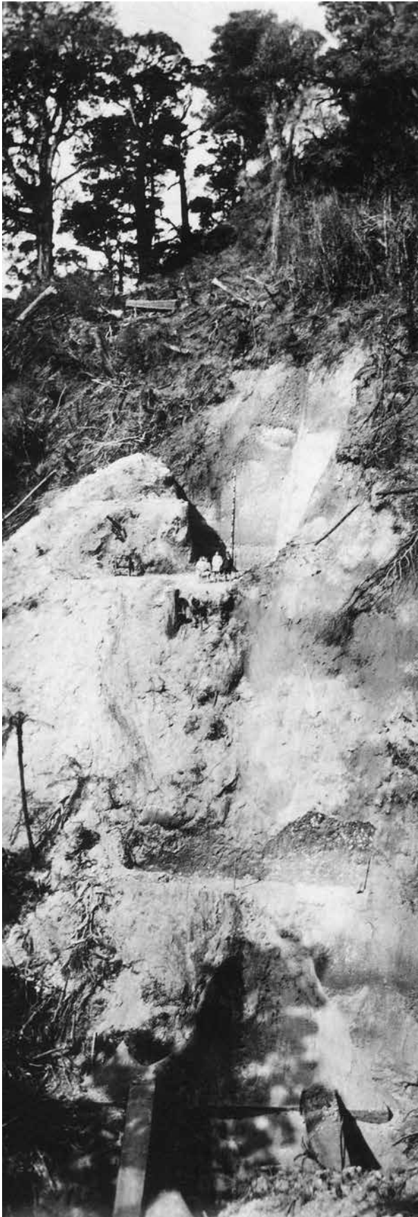
Before the tunnel could commence, a substantial bridge was necessary to cross the gully. In this photo, the work on the far bank of the gully is visible. This was the preparation for the foundations of the bridge and the digging of the tunnel. This work started in 1922. The bridge built was 120 feet long and 80 feet high.
