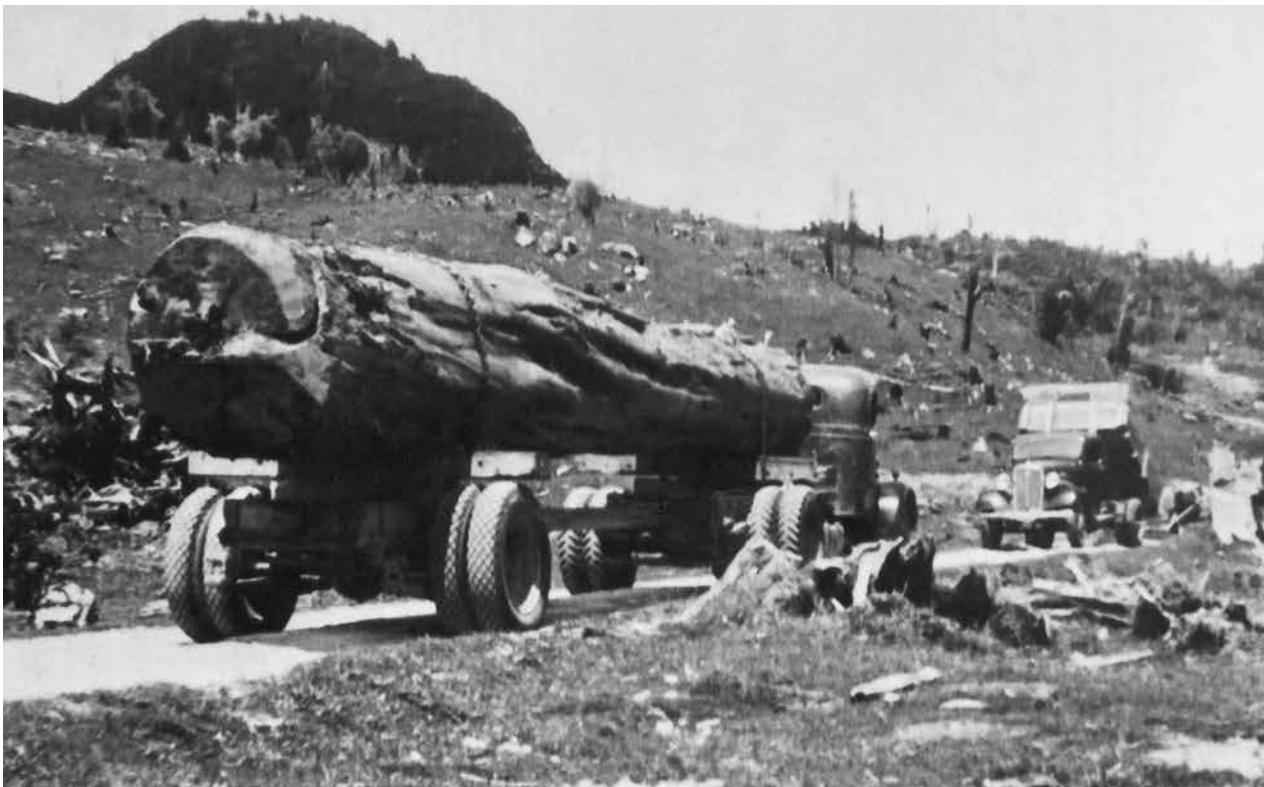
That's an extra large load for single axles! The hard working 1938 Bedford is obviously overloaded as it approaches the Company's 1935 Chevrolet on maintenance work on the Meringa-Waituhi Deviation. This logging truck was not registered for the road as its job was to save wear and tear on tractor by hauling logs from Eastward Road to a nearby skidway for transfer to the tram.
