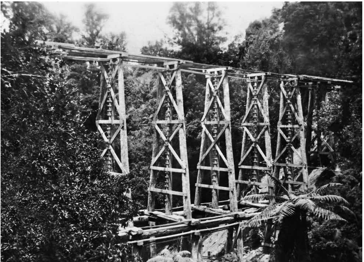
In this view the upper bents are all in place and there remains only the installation of the stringers between the three bents to the right of the photo. Frank Ward had no fear of heights and scrambled around these bridges like a spider.
