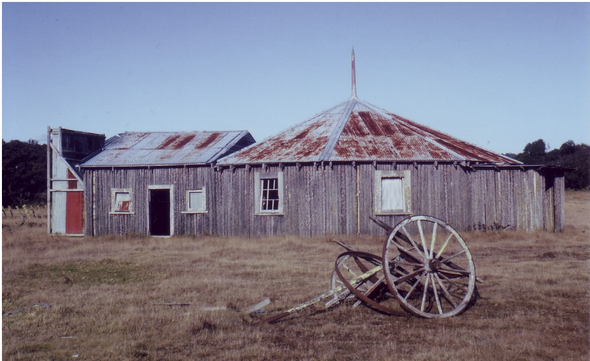
This is the dining room and kitchen built on the site later, to which E&B contributed. At the time of writing this history, Rereahu people have renovated this building to its former glory. Photo courtesy Newman Jones, Blockhouse Bay Auckland.
