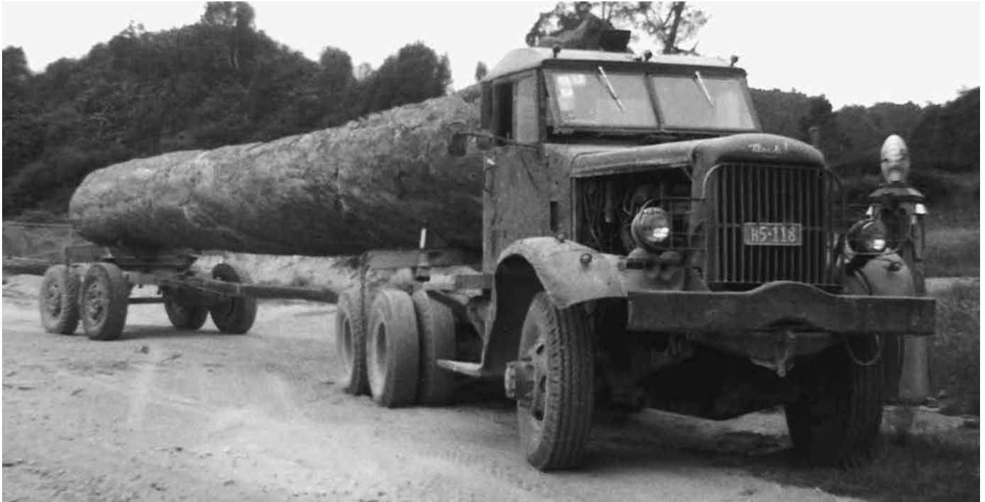
Trevor Masters also had an ex-Army Mack NM-8 model working at Ohura which is pictured here with a single large log by the petrol pump “up the Mangakara” when Ben Uncles took this photo around 1959. Ross Hopkins adds that the Mack was classed as a 6-ton 6x6 and were produced between 1944 and 1945. His eagle eye spotted the extended front hubs which told him the front diff was a banjo-type as opposed to a split housing design. He also commented on the light jinker with its single wheels and extended trailer pole.
